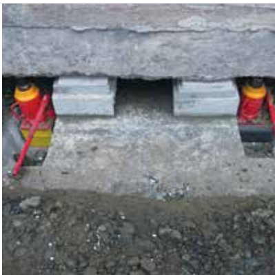
04: Jacked and supported foundation.
