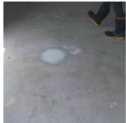
06: DPM reinstated and concrete slab core holes sealed.
