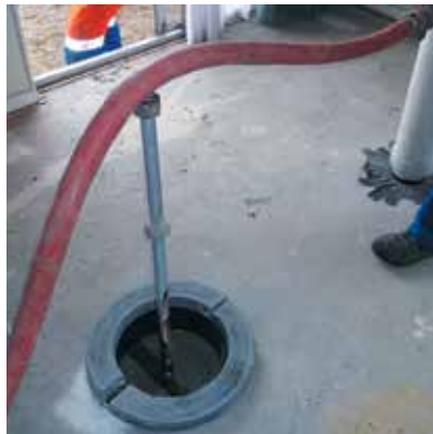
05: Concrete slab lifted at same time as foundation. Void fill poured.
