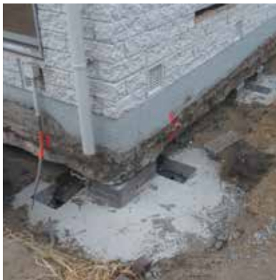
01: Entire foundation packed and jacks removed for void fill
